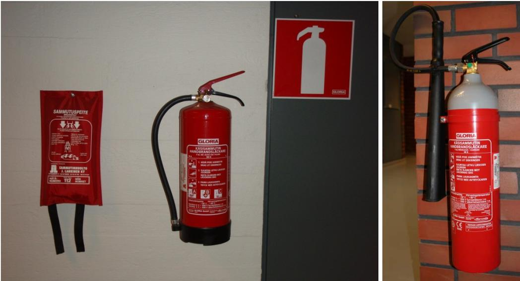
Figure 31 Fire blanket, dry chemical and CO<sub>2</sub> extinguisher.
