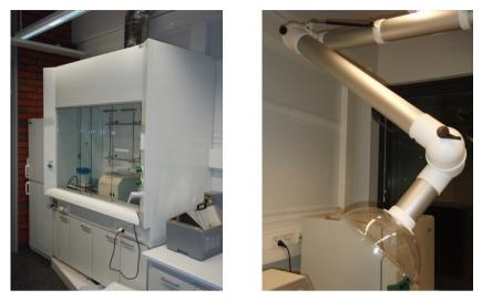
Figure 21 Vapour hood and local exhaust ventilation
