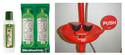
Figure 29 Eye wash bottles and eye wash station.
