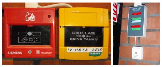
Figure 30 Fire alarm button, ventilation system "emergency stop" button and fire door control centre.
